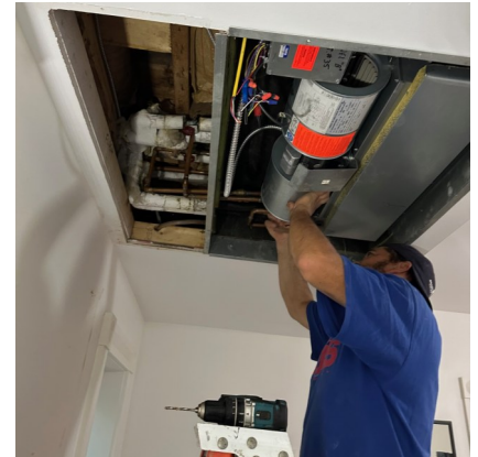
2024 Pre-Season HVAC Work at Catholic House
