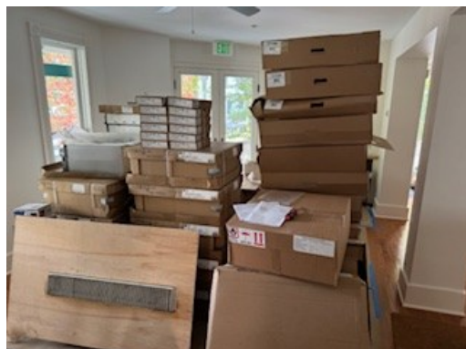
New HVAC components delivered to Catholic House
